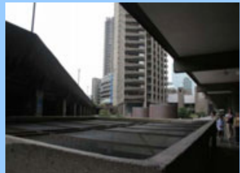
Hard to treat high rise block in an urban centre
