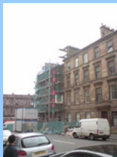
Tenement undergoing renovation, Glasgow
